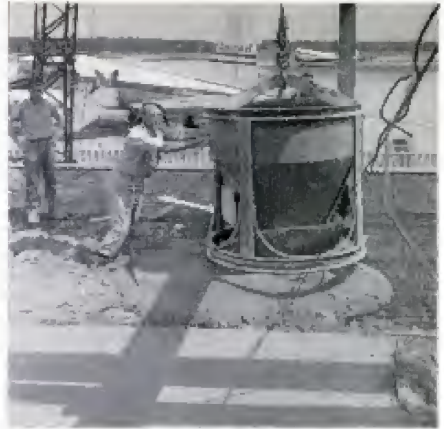
Perlite concrete poured over metal lath becomes lightweight roof deck and insulation for hangar
